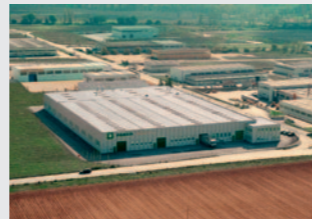
Faber S.p.A. Tecnodomus Plant Fabriano/Italy
