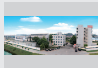
Franke (China) Kitchen Systems Co., Ltd Franke Kitchen Systems Heshan City/PRC
