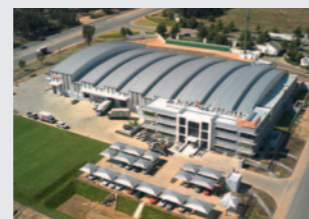
Franke Water Heating Systems (Pty) Ltd Midrand/South Africa
