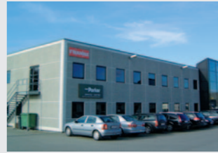
Franke KS Denmark Tilst/Denmark
