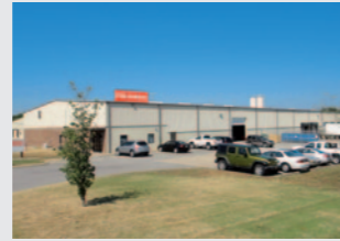
Franke Beverage Systems Inc. La Vergne, TN/USA
